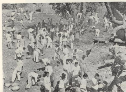
A General View The Tuck-Shop (under construction) is in the background
